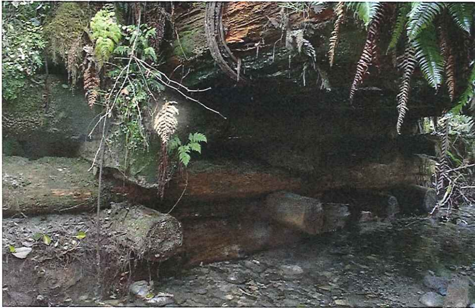
CK2265 Right Abutment
