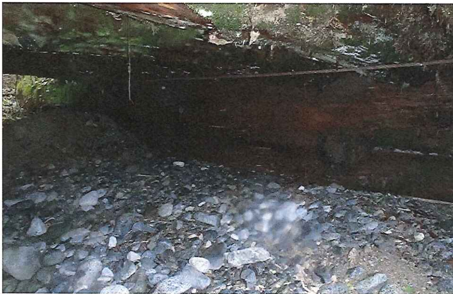
CK2265 Left Abutment
